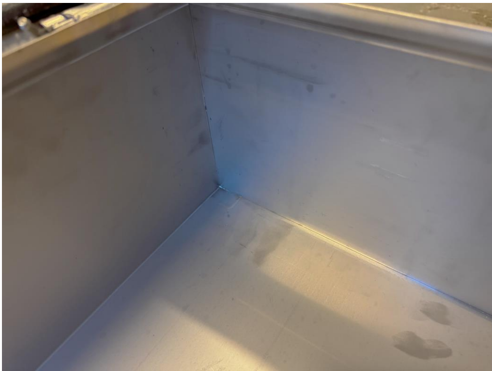
Photo 17 Visual inspection, IPX6. No ingress of water observed.
